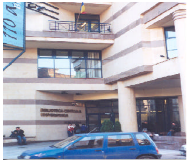
The new entrance to the Central University Library.
