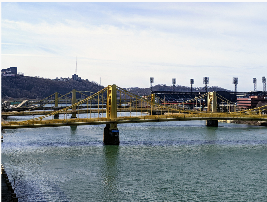
The Three Sisters suspension bridges in Pittsburgh, PA.
