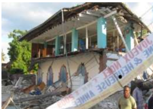
The public library in Petit Goâve after the 2010 earthquake.
