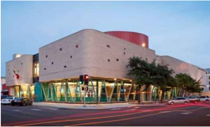
The Stephens Central Library in San Angelo, Texas, took over a vacant downtown department store building. Photo by Tom Kessler.
